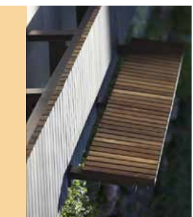
Fig. 7.3.119 Timber Bench Seating
