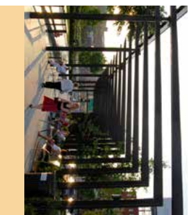
Fig. 7.3.127 Bespoke Shelter: Powdercoated Aluminium
