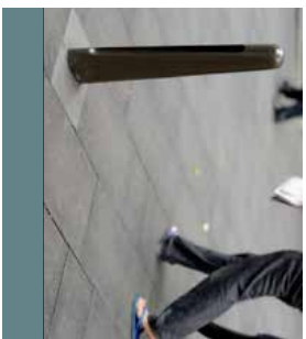
Fig. 7.3.121 Bollard: Bronze Powdercoated Aluminium
