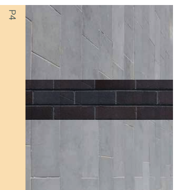
Fig. 7.3.114 Hamlet Blue Brick with COS Concrete Unit Paver
